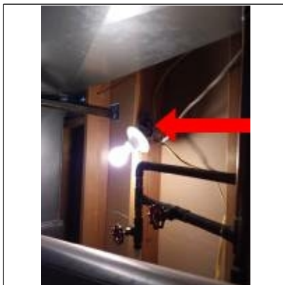
Exposed wiring
