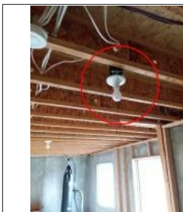
Exposed wires
